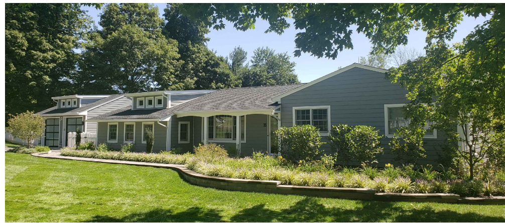
2 PICTURE 2 FRONT RIGHT VIEW (MORRISTOWN RD) SCALE: NTS
